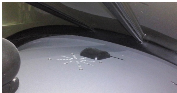
Figure 34-005 GA 26C GPS antenna installation
