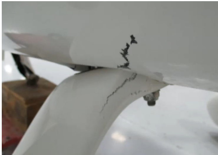
Figure 53-001 Example of fuselage main frame damage
